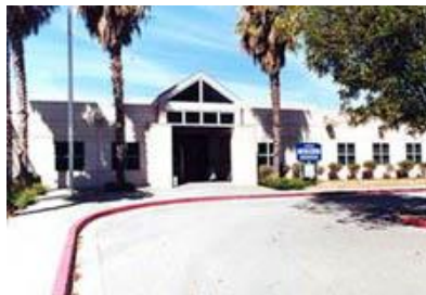
Elmwood Correctional Facility for Women 701 S. Abel St. Milpitas, CA 95035
